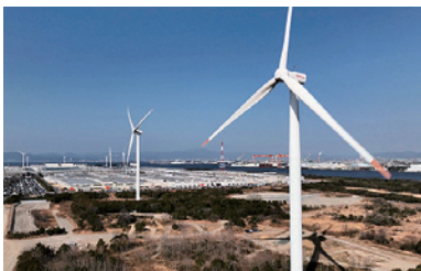
Tahara wind power generation
