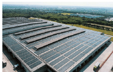
Solar panels installed at TMMIN
